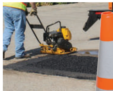
Vibrating plate compacts the mix.
