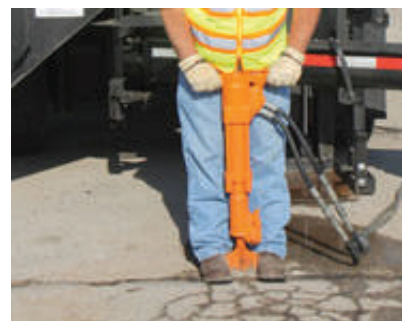
Uniform edges are cut with a pavement breaker.
