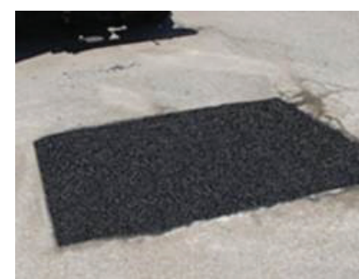
Perfect pothole patch: years of protection!
