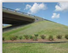
Transportation Gateway Improvements
