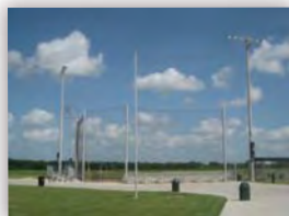
Seabourne Creek Regional Sports Complex Lighting
