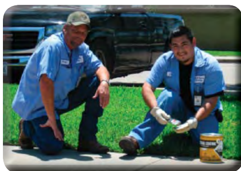
Installing RDC Funded Mile Markers Pictured (L-R): Public Works, Street Division Employees: Darryl Lindemann and Leroy Lopez.
