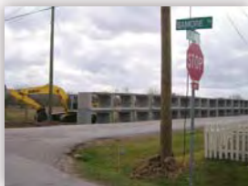
Bamore Road Reconstruction Project
