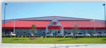
National Oilwell Varco Relocation
