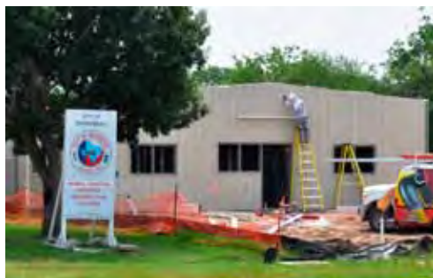
Crews work on the facade of the new Animal Control Facility.
