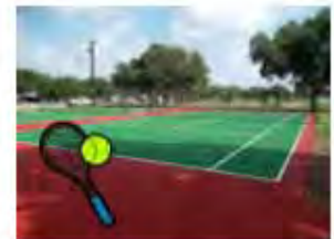
Sunset Park Tennis Court Improvements
