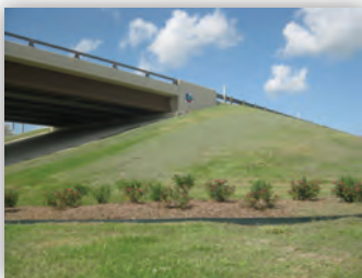
Transportation Gateway Improvements
