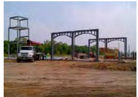
Steel girders for vehicle bays and front entry tower at Fire Station No. 3.
