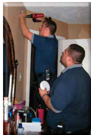
Firefighter Daryl Ustynik and George Velasquez, Jr. install a smoke detector in the home of Hortencia Rangel. The device is provided at no charge as part of RFD's Baby Safe program.
