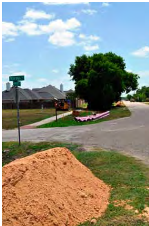
Purple reclaimed water pipe lays along Airport Avenue awaiting installation.
