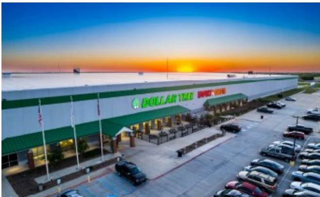
Dollar Tree Distribution Center
